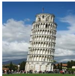
Leaning tower of Pisa
